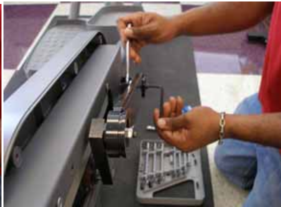
Fig. 8: installing the new control link assembly
